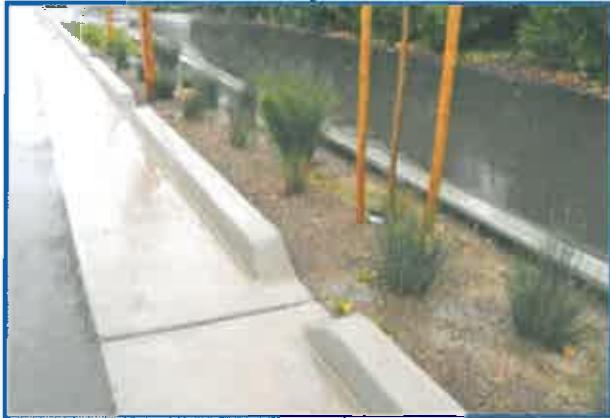
Curb cuts along Rosita Ave. help direct stormwater to a bioswale. Photo credit: Gary Hedden
