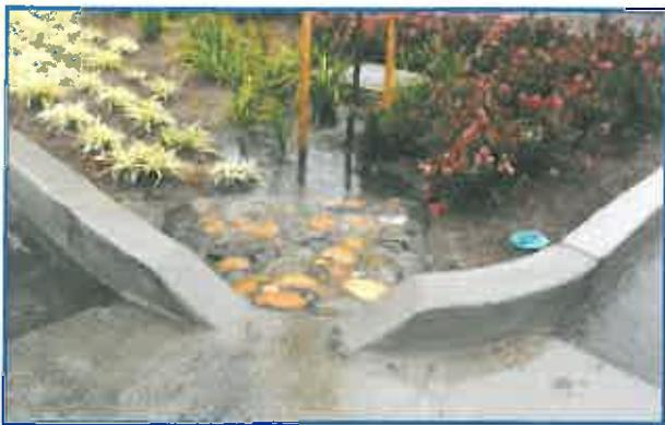
Rocks and special soil in the swale help to slow and sink the stormwater. Photo credit: Gary Hedden
