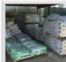
Outdoor materials stored on pallets and covered.
