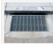
Only rain down the storm drain.
