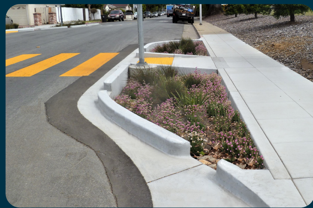
▲ This GSI project captures and treats stormwater from a public street.
