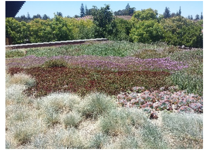
Figure 2-7 Green Roof, David and Lucille Packard Foundation Headquarters (Source: City of Los Altos)
