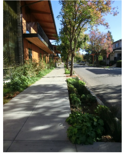
Figure 2-11 David and Lucile Packard Foundation curbside flow-through rain garden (Source: EOA, Inc.)
