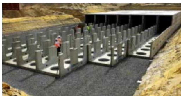
Figure 2-9 Subsurface vault under construction (Source: Contech)
