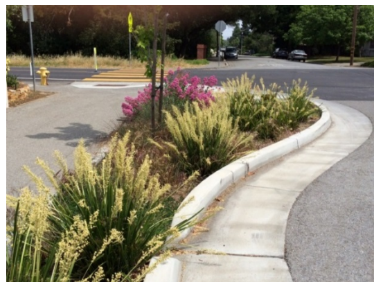
Figure 2-2 Stormwater curb extension, Rosita Park, Los Altos (Source: City of Los Altos)
