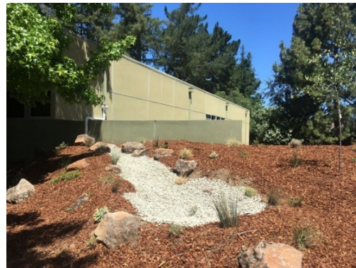
Figure 2-12 Woodland Branch Library bioretention area and rain garden (Source: City of Los Altos)
