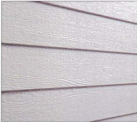
FIRST LEVEL EXTERIOR: HORIZONTAL WOOD SIDING - LIGHT GREEN COLOR
