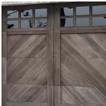
Stained garage and front door
