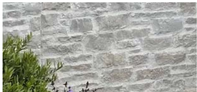
Stone base at facade
