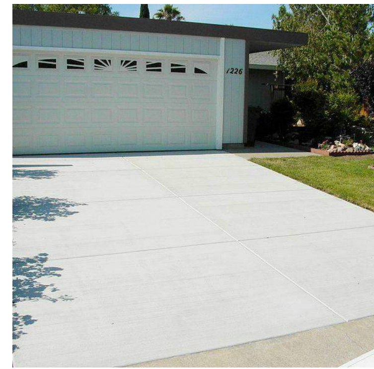
CONCRETE DRIVEWAY & WALKWAY
