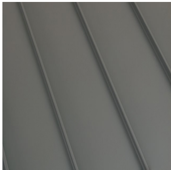
Standing Seam Metal Roof
