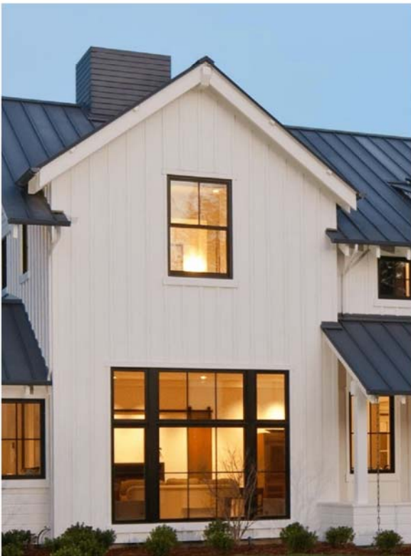
FIBERGLASS WINDOW FRAME (DARK COLOR) WITH WOOD TRIM (LIGHT COLOR) MANUF.: MARVIN OR SIMILAR
