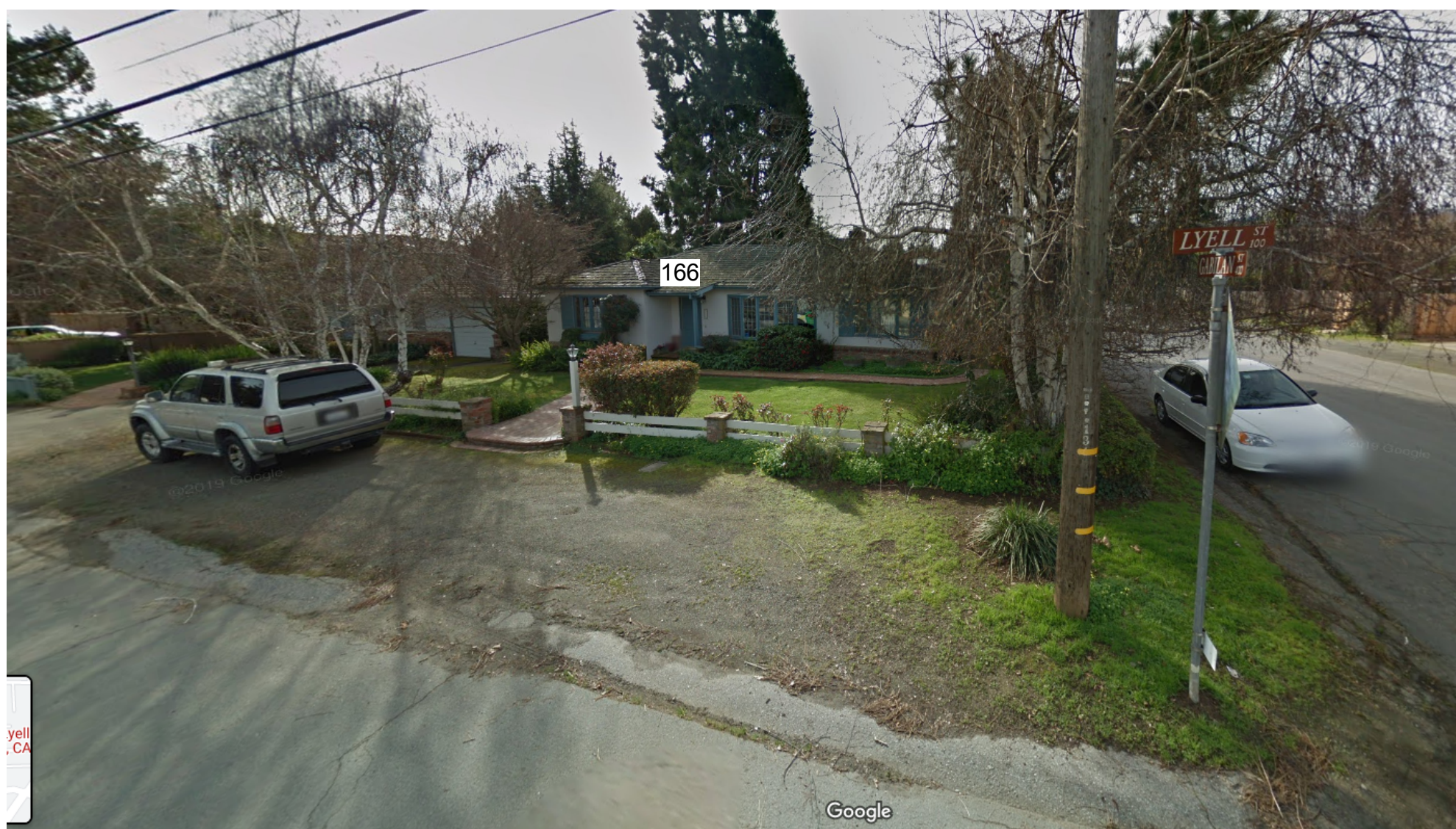
VIEW LOOKING OF 166 LYELL STEET EXISTING HOUSE
