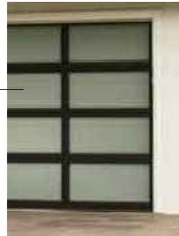
GARAGE DOOR: DARK ALUMINUM FRAME WITH ETCHED GLASS
