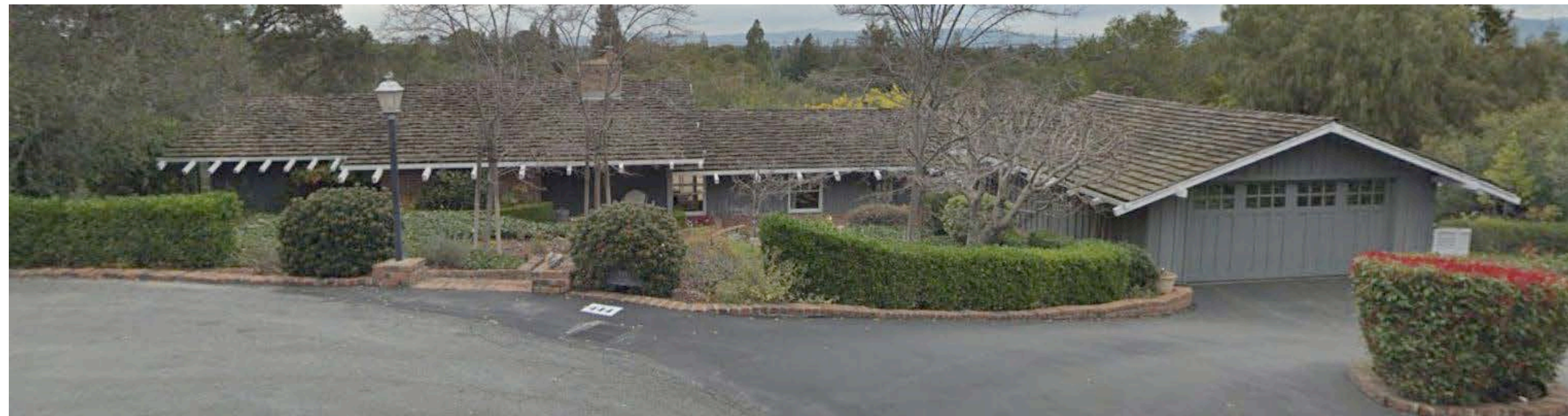
444 FIR LANE - EXISTING ELEVATION FROM STREET
