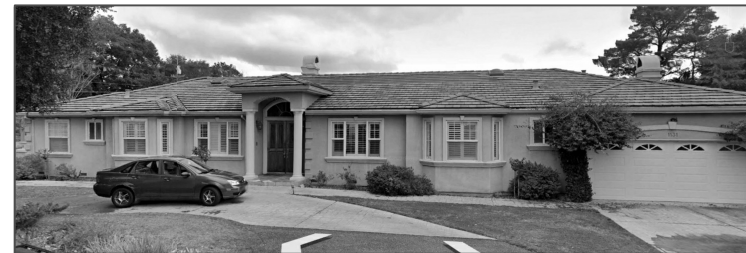
1131 PAYNE DRIVE ONE STORY ARCH STYLE: MEDITERRANEAN MATERIALS: WALL: STUCCO AND STONE TRIMS ROOF: CONCRETE TILE DRIVEWAY: PERMEABLE STONE GARAGE LOCATION: FRONT
