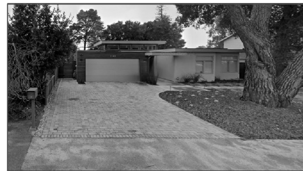
1141 PAYNE DRIVE ONE STORY ARCH STYLE: EICHLER MATERIALS: WALL: STUCCO AND WOOD SIDING ROOF: TAR AND GRAVEL DRIVEWAY: PERMEABLE STONE GARAGE LOCATION: FRONT
