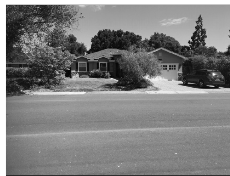
1135 LISA LANE ONE STORY ARCH STYLE: BUNGALOW MATERIALS: WALL: STUCCO/ STONE VENEER ROOF: COMPOSITION SHINGLE DRIVEWAY: PERMEABLE STONE GARAGE LOCATION: FRONT
