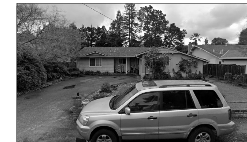
1150 PAYNE DRIVE ONE STORY ARCH STYLE: AMERICAN CRAFTSMAN MATERIALS: WALL: WOOD SIDING/ BOARD AND BATTEN ROOF: COMPOSITION SHINGLE DRIVEWAY: CONCRETE GARAGE LOCATION: FRONT/SIDE ACCESS
