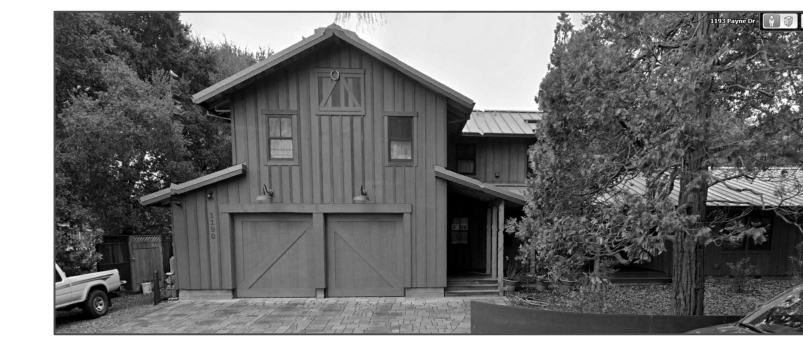
1190 PAYNE DRIVE TWO STORY ARCH STYLE: FARMHOUSE WALL: BOARD AND BATTEN ROOF: METAL DRIVEWAY: CONCRETE GARAGE LOCATION: FRONT
