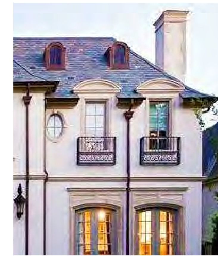
7. SIDE WING W/ HIPPED ROOF, ARCHED WINDOWS BREAK ROOF EAVES, HORIZONTAL TRIM BAND, DOWNSPOUTS WITH COLLECTORS
