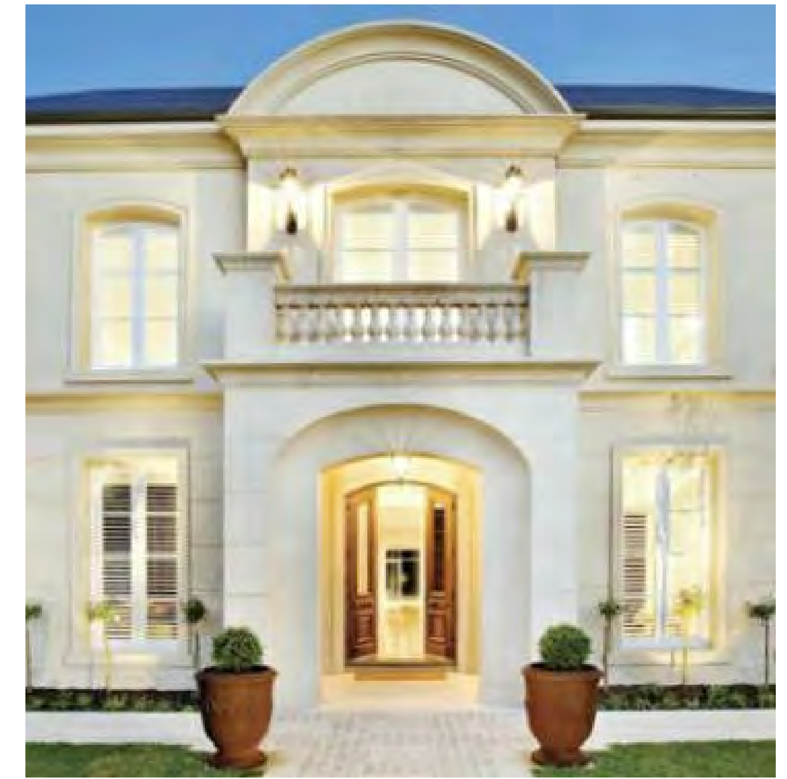
3. LIMESTONE BALCONY OVER ENTRANCE & STUCCO SIDING
