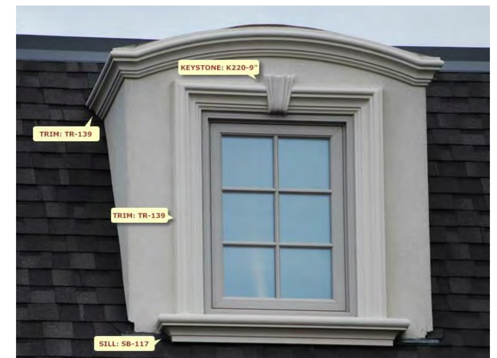
1. WINDOWS WITH TRIM
