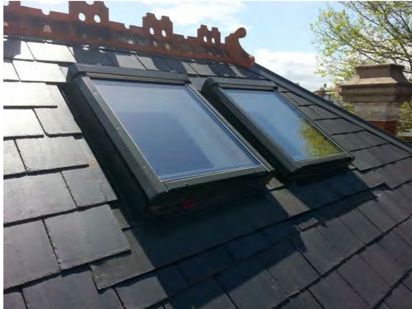
17. SLATE ROOF WITH SKYLIGHTS
