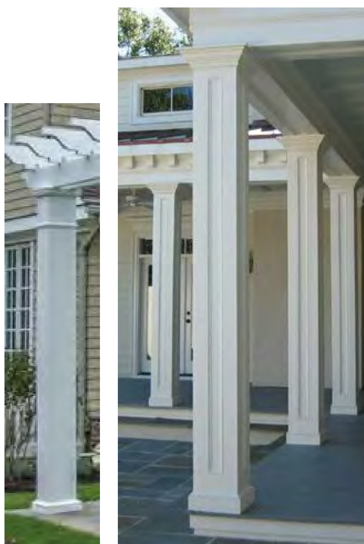
4. SQUARE COLUMNS AT REAR TRELLIS
