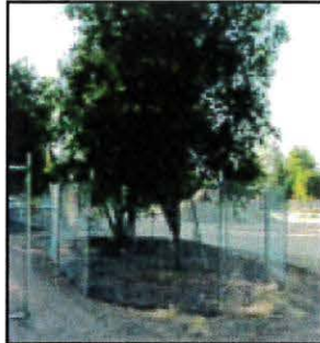
IMAGE 2.15-1 Tree Protection Fence at the Dripline
