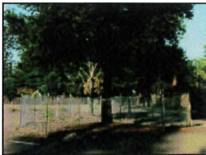
IMAGE 2.15-2 Tree Protection Fence at the Dripline
