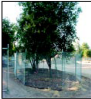
IMAGE 2.15-1 Tree Protection Fence at the Dripline
