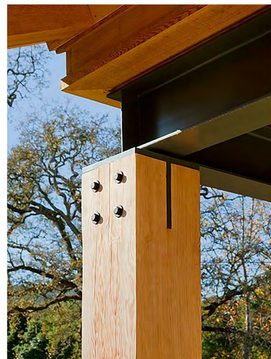
PORCH COLUMN AND BEAM
