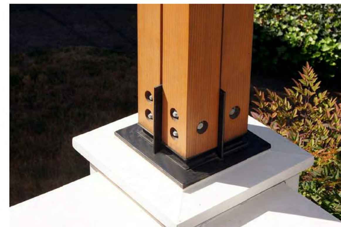
PORCH COLUMN BASE
