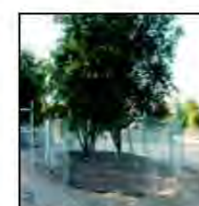
IMAGE 2.15-1 Tree Protection Fence at the Drip-line
