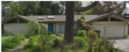
133 SOLANA DRIVE (1-STORY RESIDENCE)
