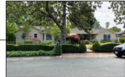
169 DOUD DRIVE (1-STORY RESIDENCE)
