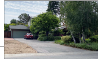
149 DOUD DRIVE (2-STORY RESIDENCE)
