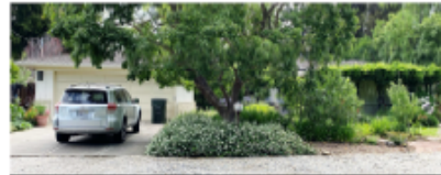
147 SOLANA DRIVE (1-STORY RESIDENCE)
