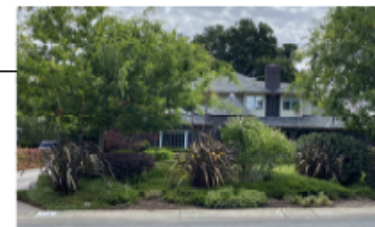
115 DOUD DRIVE (2-STORY RESIDENCE)
