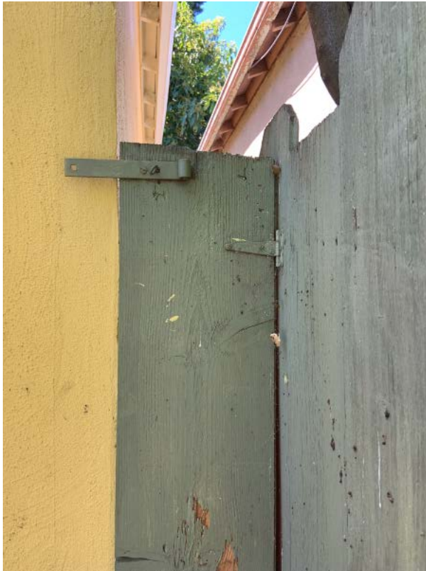
Gate used for maintenance between Accessory Building and Garage
