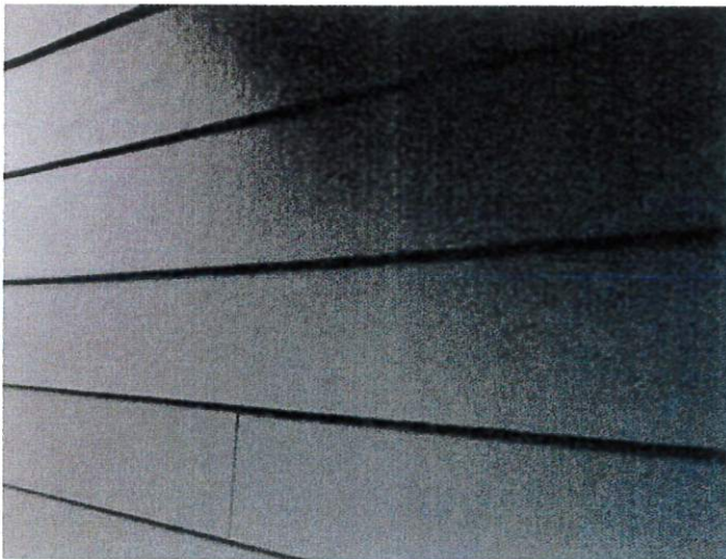
Horizontal Siding Material - Hardie Artisan V Rustic - painted
