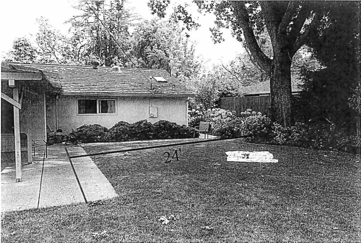
Image #3 – Tree T2 – valley oak. Approximate location of new foundation (red line) and minimum distance to base of valley oak trunk.
