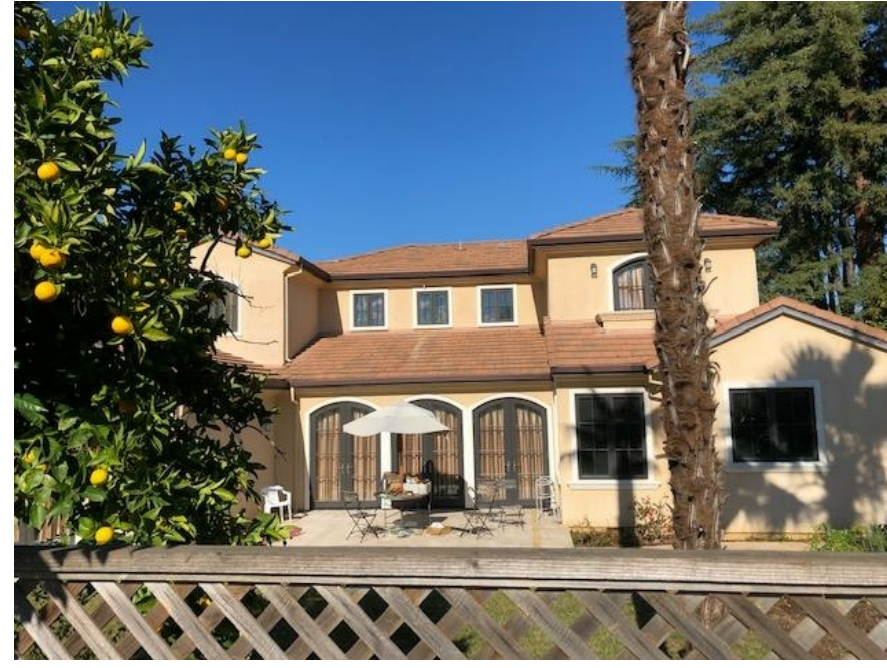
1442 MORTON AVE. BACK OF HOUSE AS SEEN FROM 1798 WENRICK COURT.
