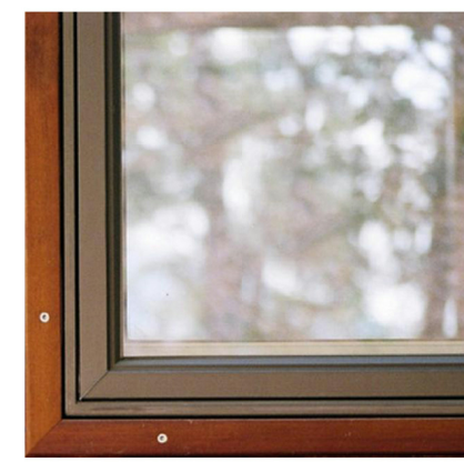
Trim Detail - Redwood Semi Transparent (Alt Western Cedar Redwood stain)
