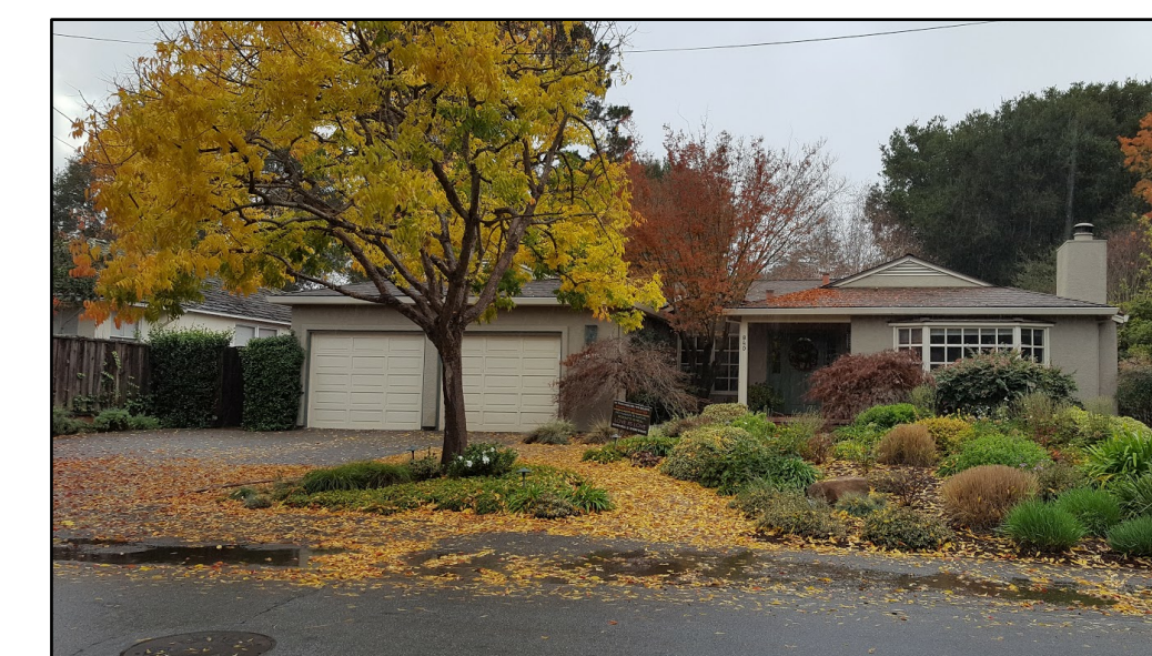
EXISTING HOUSE AT 840 PARMA WAY
