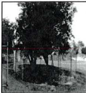
IMAGE 2.15-1 Tree Protection Fence at the Dripline
