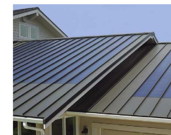
Roof Material – Standing Seam Metal – Bronze color – Custom Built Metals
