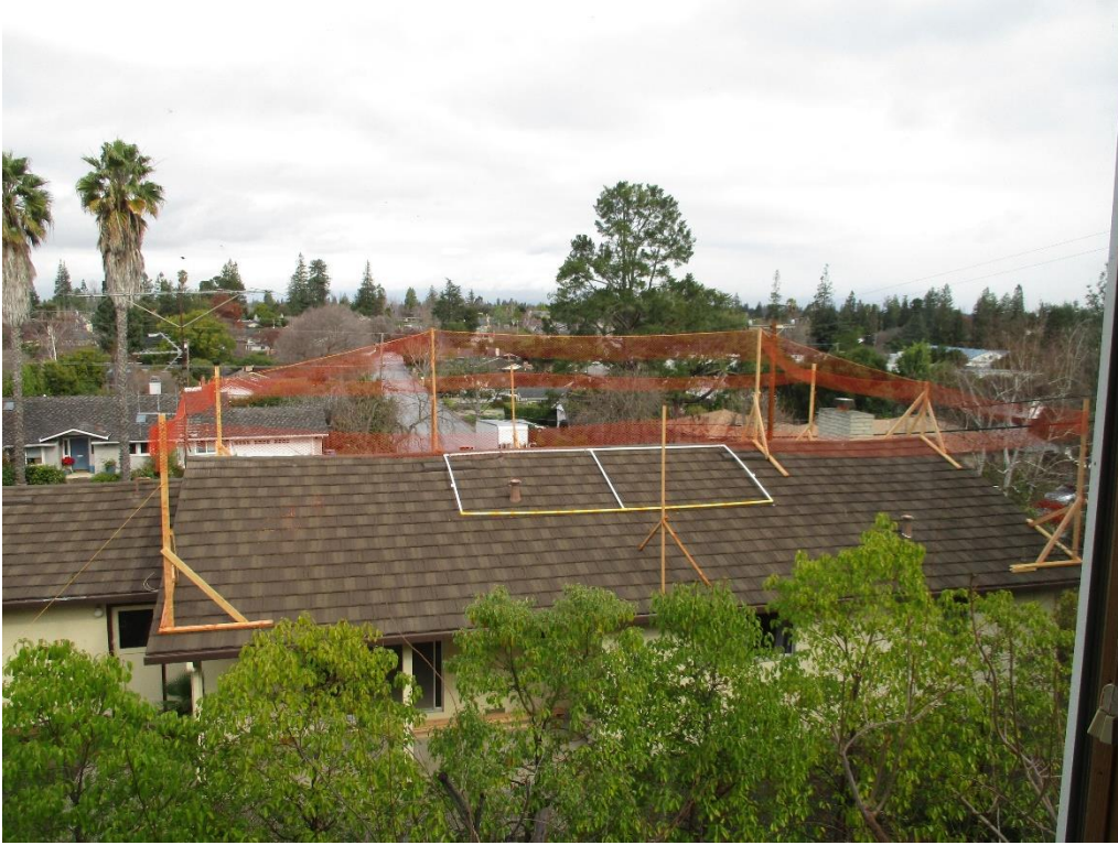
1. From bay window (approximately 48" from floor)
