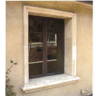
Stone Windows & Doors Trim
