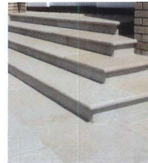
Tile Finished Concrete Steps
