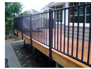
EXAMPLE OF RAILING @ LIGHT WELLS
