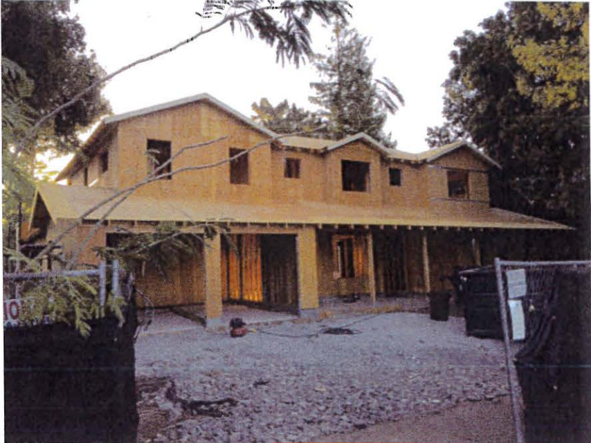
1325 Oakhurst 2 stories, 4200 sf, Craftsman with metal roof under construction
