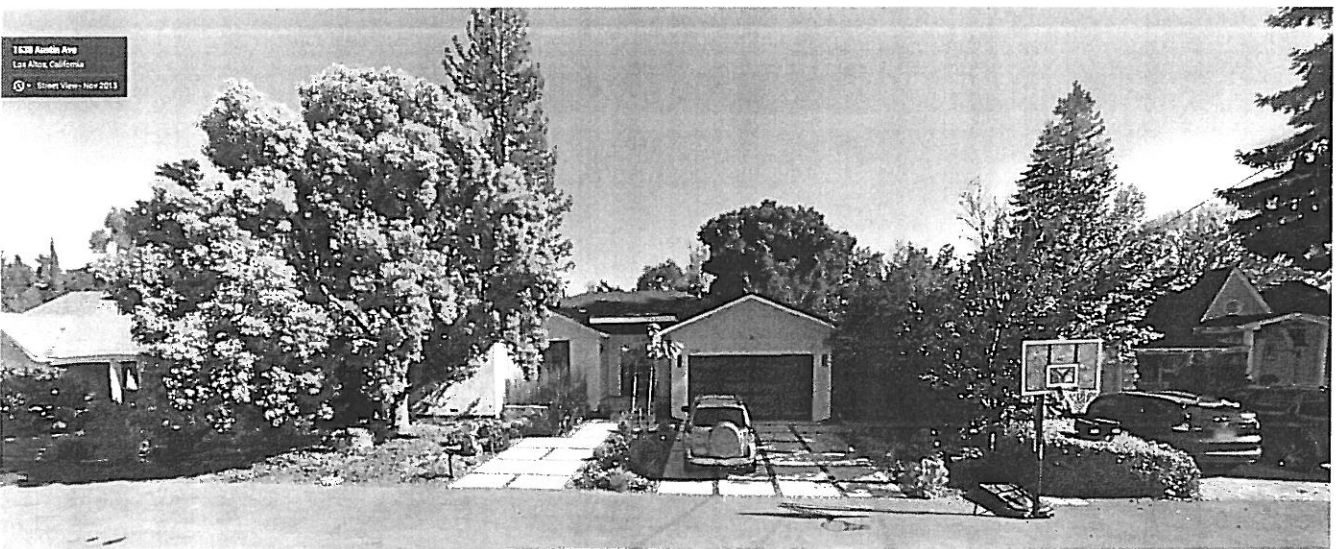
Across 1 st Right Side: 1635 Austin Avenue, 1-Story
