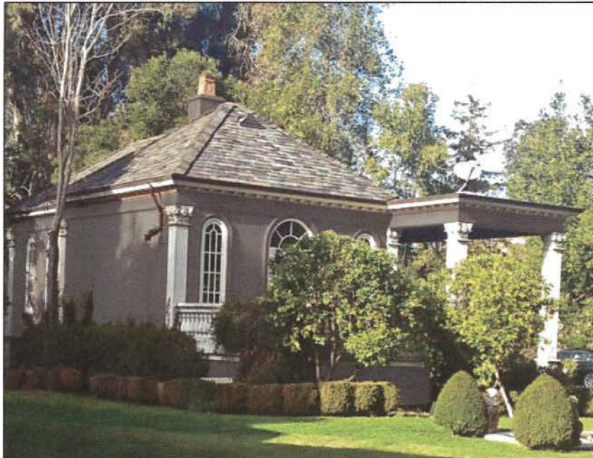
EXISTING BUILDING VIEW
