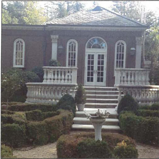
EXISTING BUILDING VIEW
