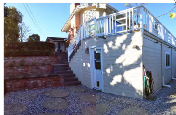
ROOF DECK AND OFFICE TO BE REMOVED
