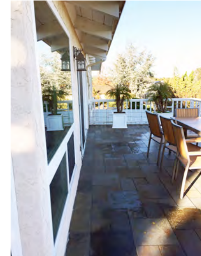
ROOF DECK TO BE REMOVED
