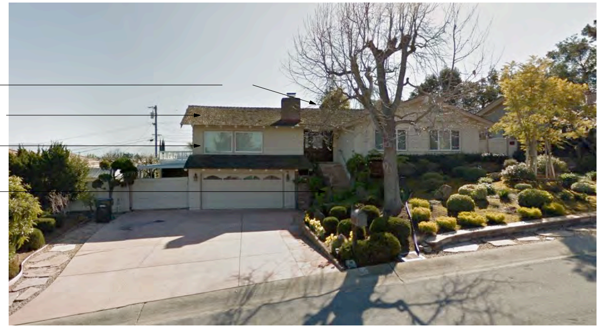
FRONT OF EXISTING HOUSE AND MATERIAL CALLOUTS
