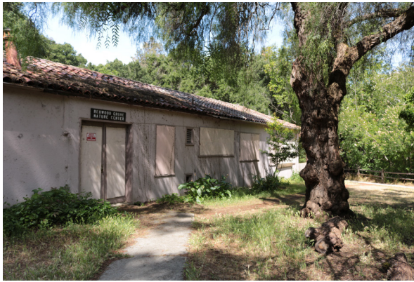
Concrete path at the east elevation (ARG, 2019).
