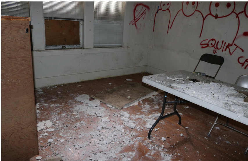
Craft room, view of floor and walls.
