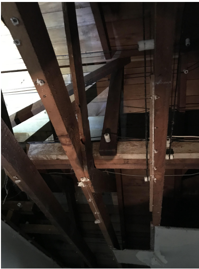
Photo #13: Roof Framing and Ridge Board at East Wing of the Building
