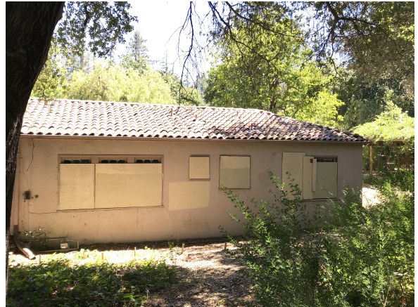
Photo #4 - South End of the West Elevation of the West Wing of the Building
