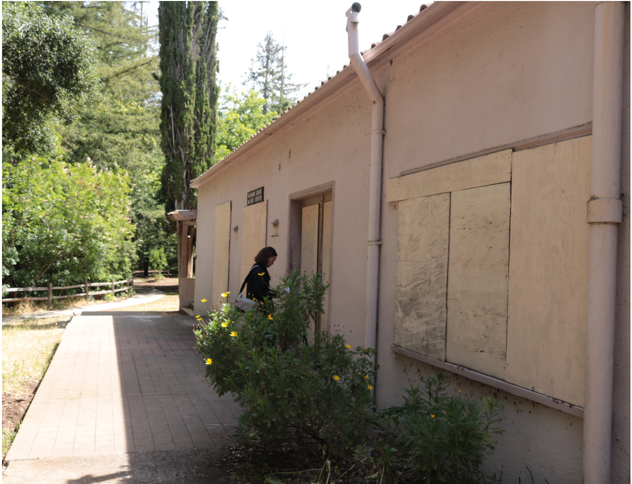
View of north elevation looking east.
