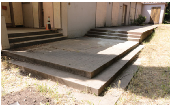
Figure 4. Concrete porch and terrace (photo: ARG, May 2019).
