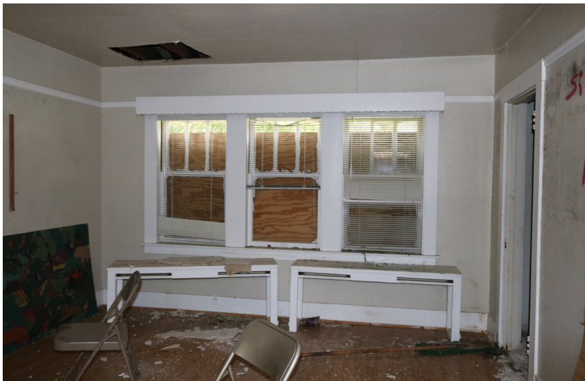
Animal room, view looking west.
