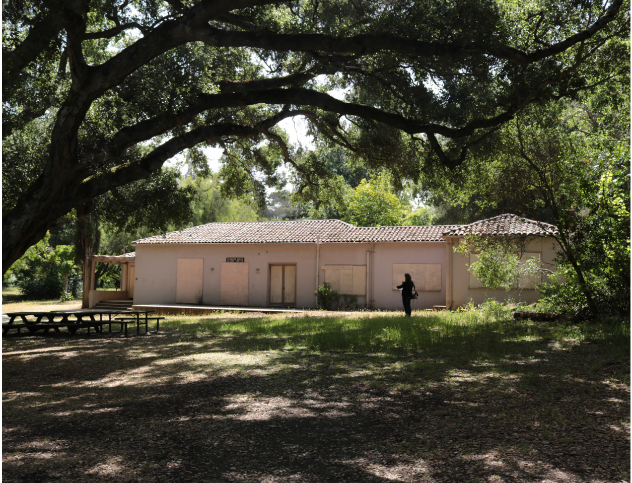
Overall view of north elevation from edge of redwood grove.
