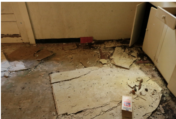
Vinyl tile in the West Kitchen (ARG, 2019).
