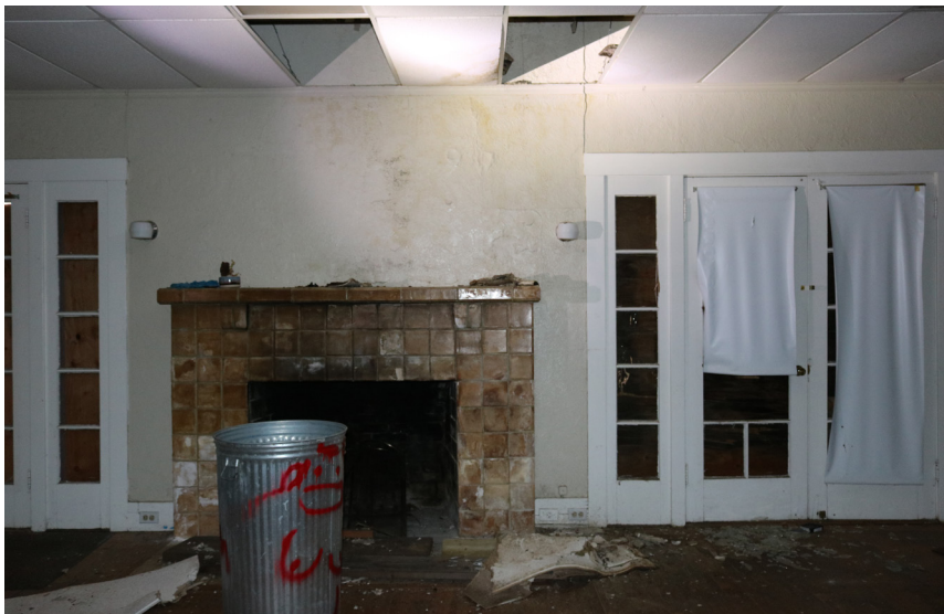
Looking south, including view of fireplace, inside main room.
