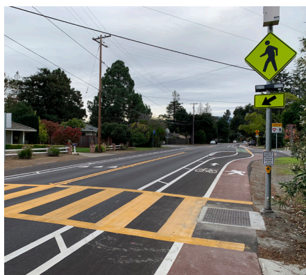
High-visibility crosswalk and Rectangular Rapid Flashing Beacon
