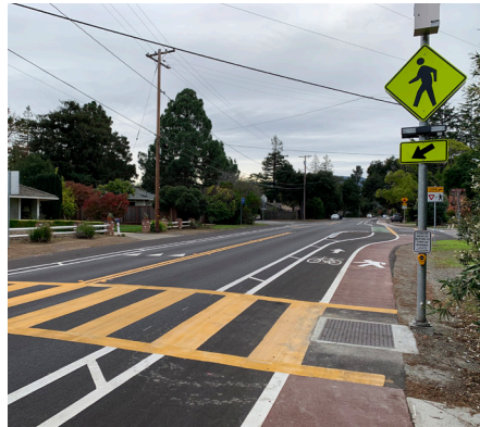
High-visibility crosswalk and Rectangular Rapid Flashing Beacon
