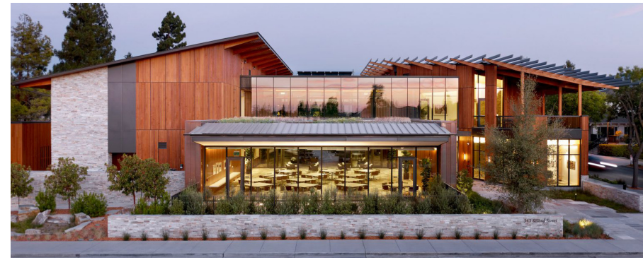
PACKARD FOUNDATION HEADQUARTER 1
