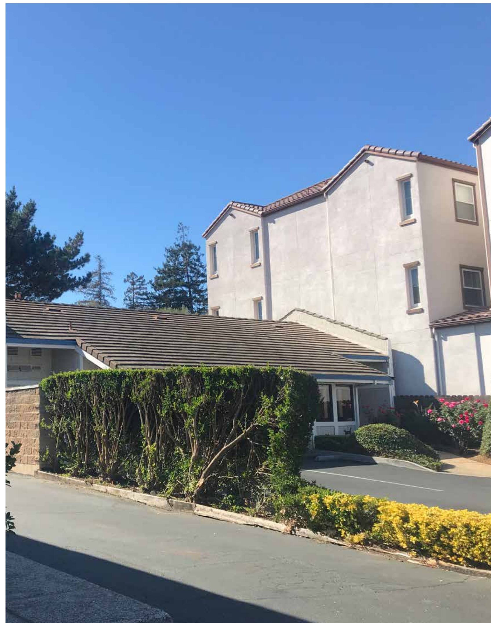
2. 440 First St and Lennar Project to the North
