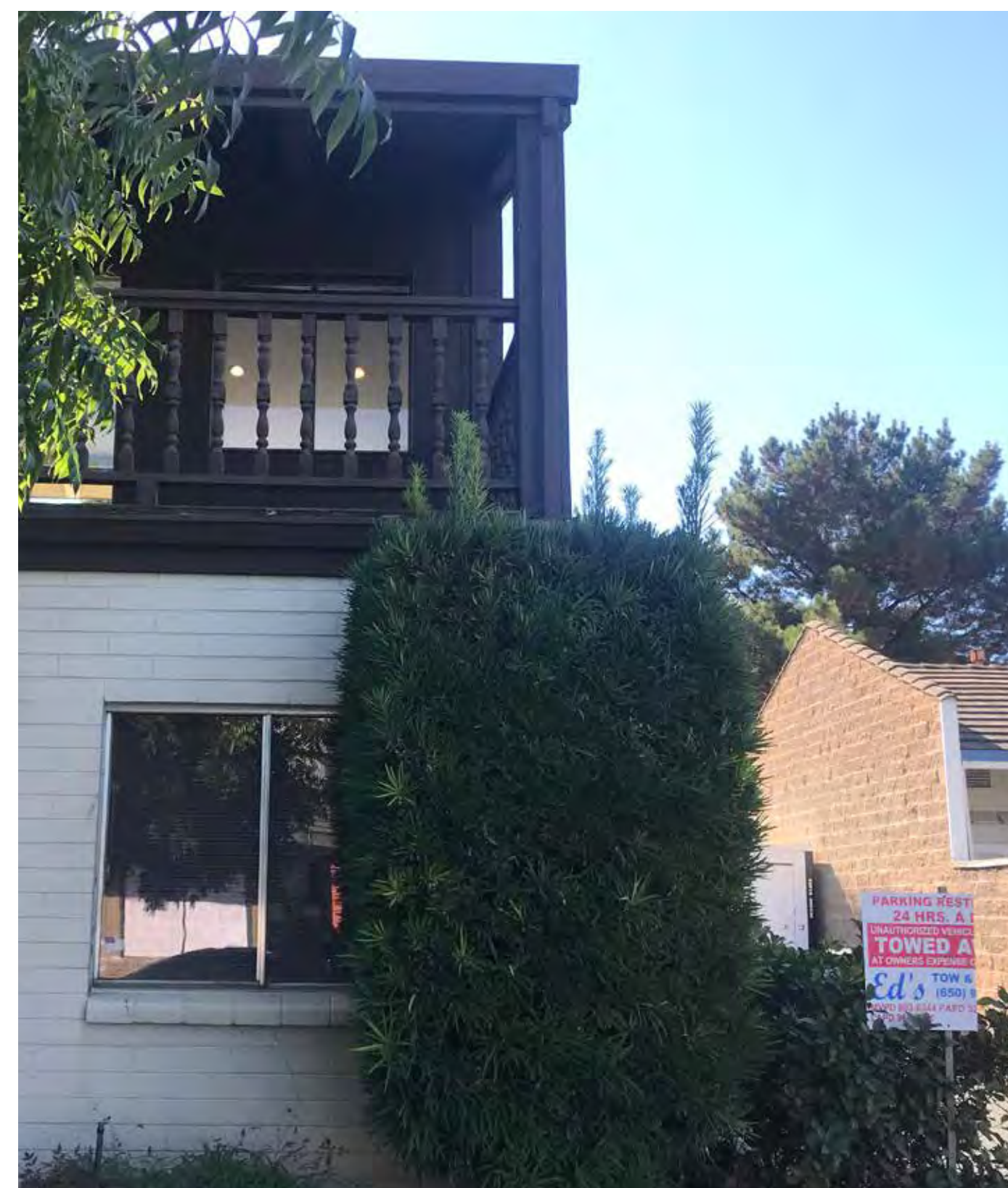
3. Existing Bldg at 450 First St
