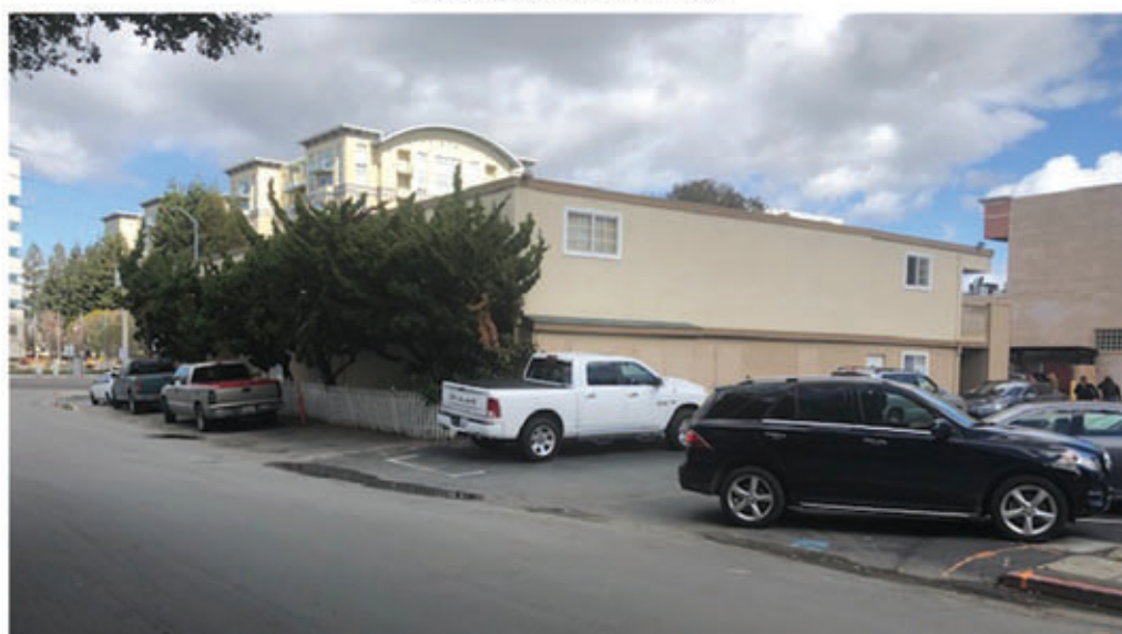
VIEW FROM JORDAN AVE. - REAR
