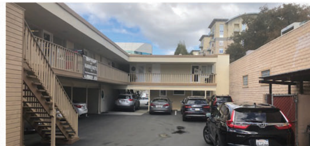
VIEW OF EAST SIDE OF BUILDING
