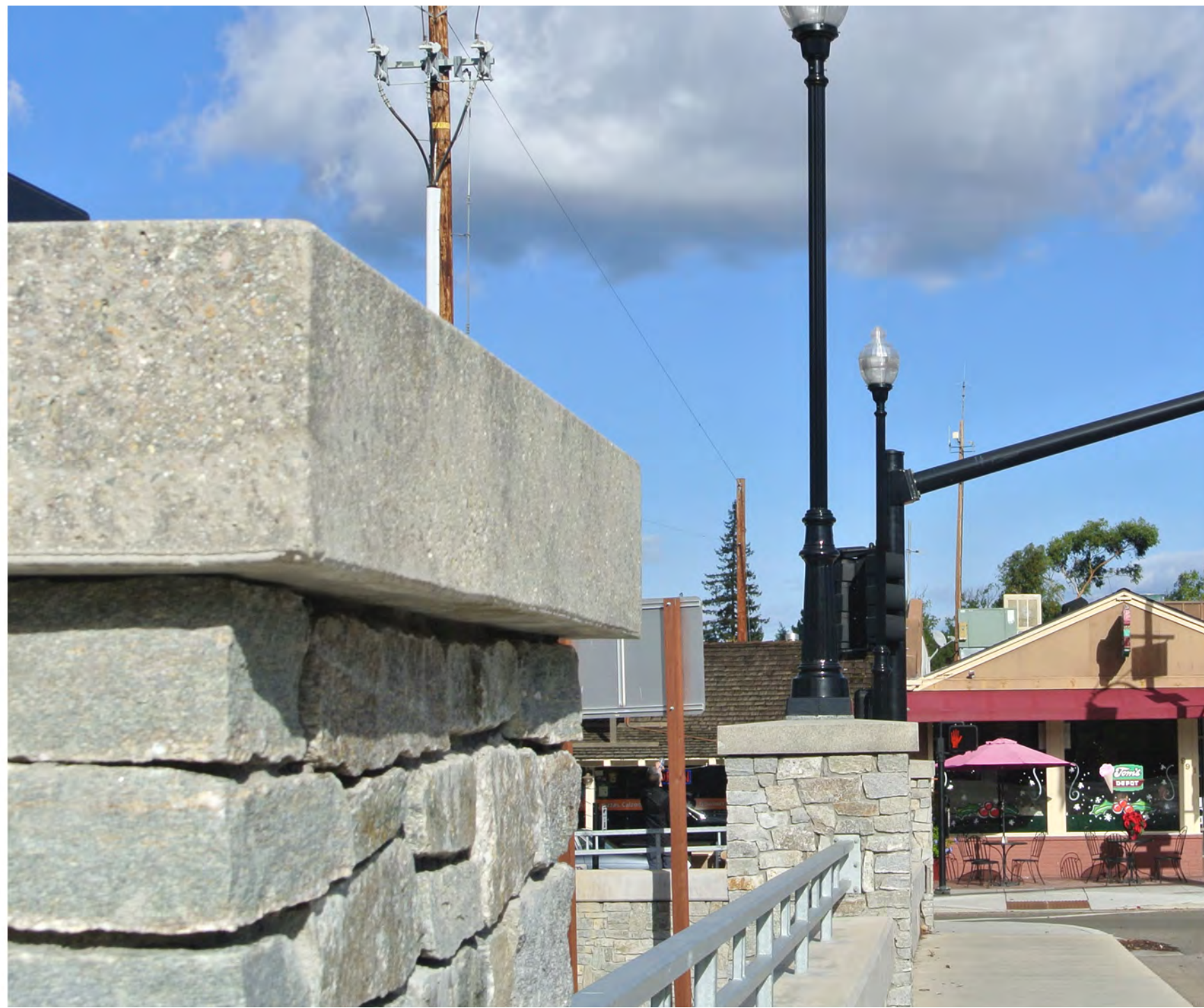
FROM BRIDGE OVER FOOTHILL EXPRESSWAY EXISTING VIEW
