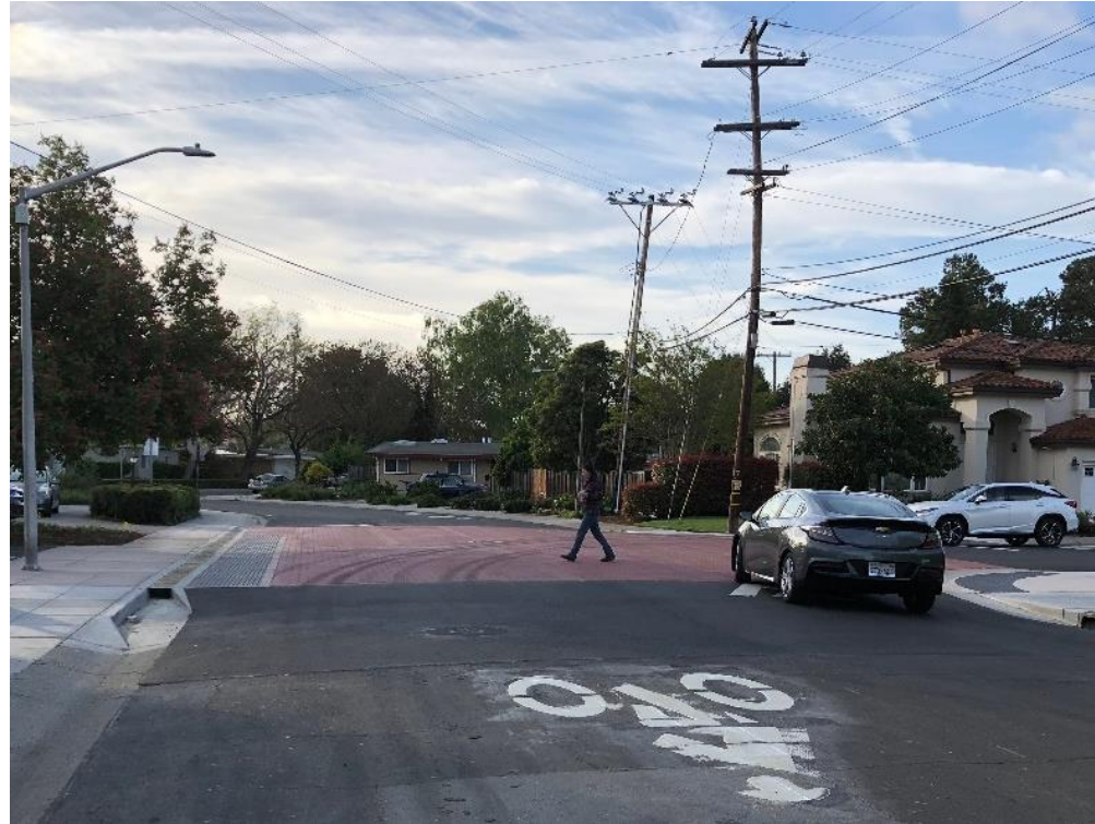
City of Palo Alto Raised Intersection (Ross Rd/Mayview Ave)
