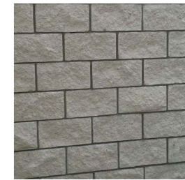
DECORATIVE MASONRY WALL
