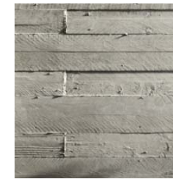
BOARD FORM FINISH CONCRETE
