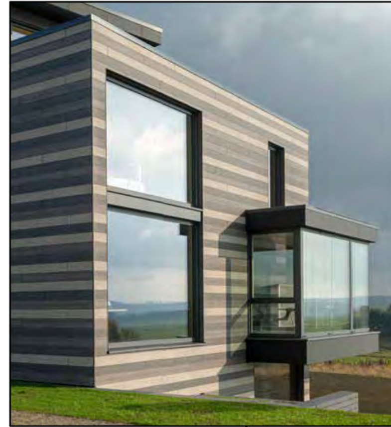
TRESPA® HORIZONTAL SIDING WITH VARIEGATED SIDING WITH SEEMINGLY RANDOM VERT. JOINTS WHERE LENGTHS WARRANT IT; NO JOINTS FOR SHORT RUNS
