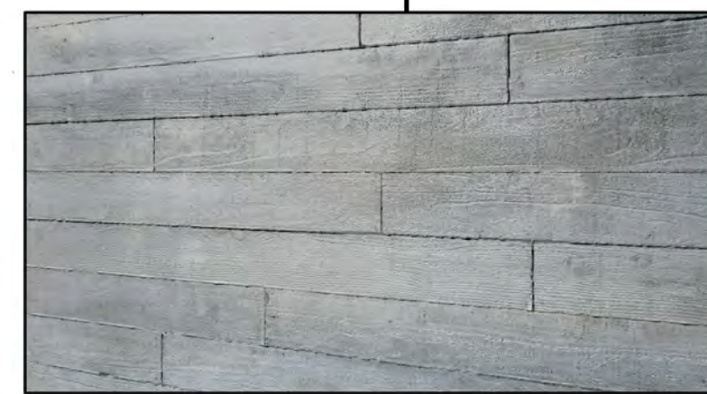
BOARD FORMED CONCRETE PATIO WALLS
