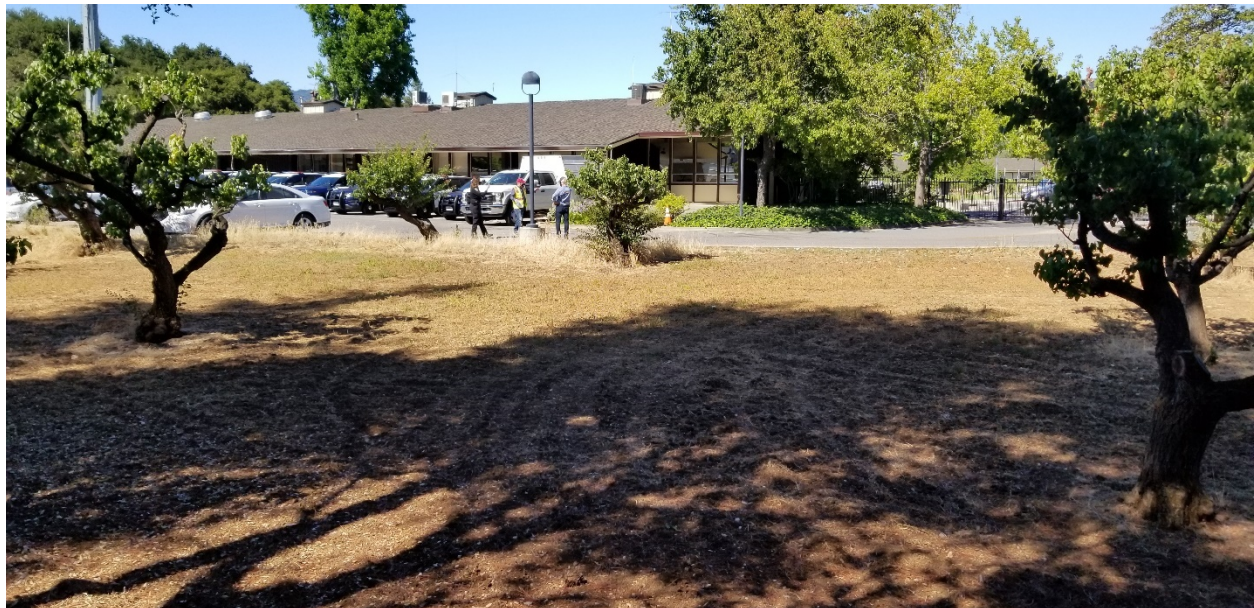
Figure 7: Looking west at police station.
