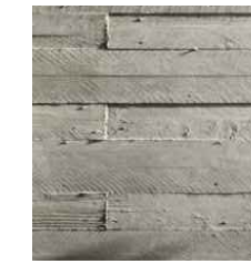
BOARD FORM FINISH CONCRETE
