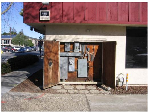
Photo 5, Electric utility meters and telephone connections (inside enclosure), and gas meter on side of building (to right of enclosure).
