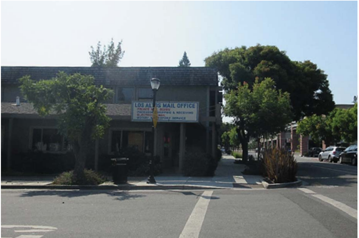
Viewing southeast towards the northwest corner of the site from Shasta Street.
