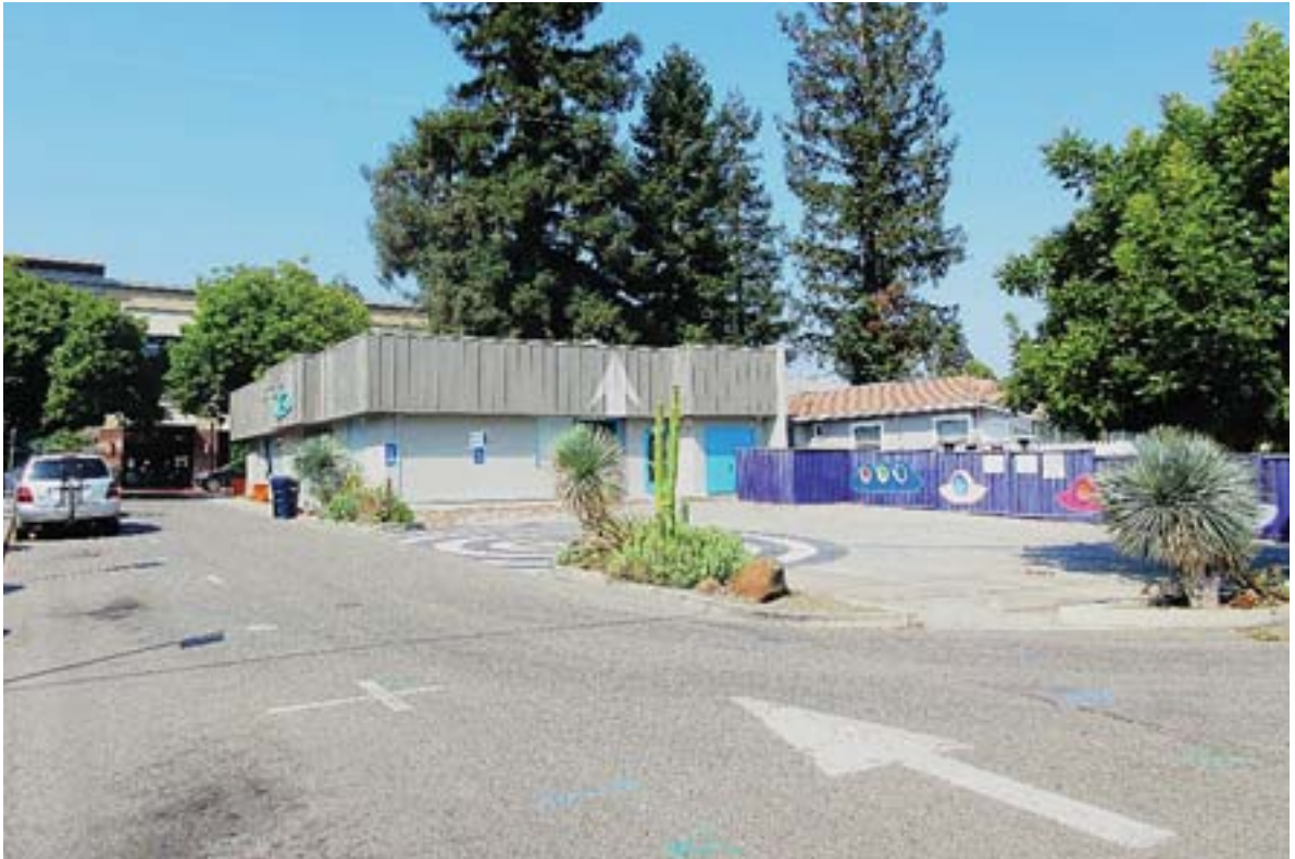
Viewing west towards the southeast corner of the site from Plaza North.
