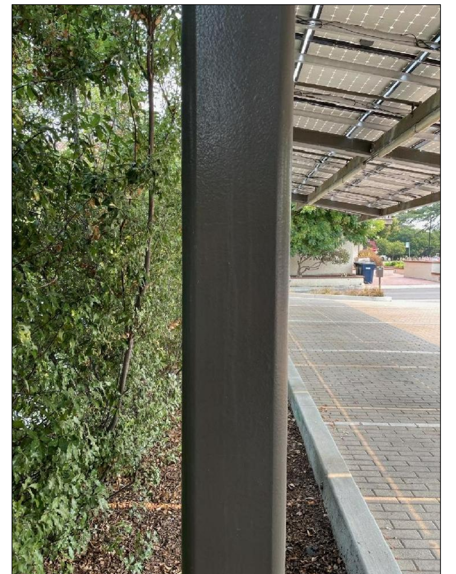
EXISTING PACKARD FOUNDATION PARKING LOT AT 323 2ND STREET: RECTANGULAR STEEL TUBE COLUMN
