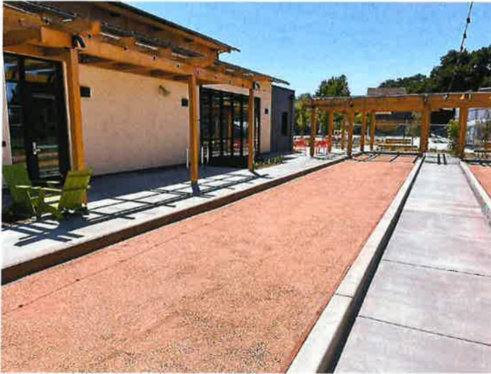
Exterior at Bocce Courts
