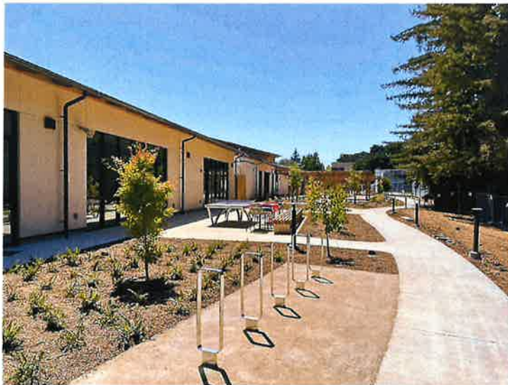
Exterior at Teen Patio
